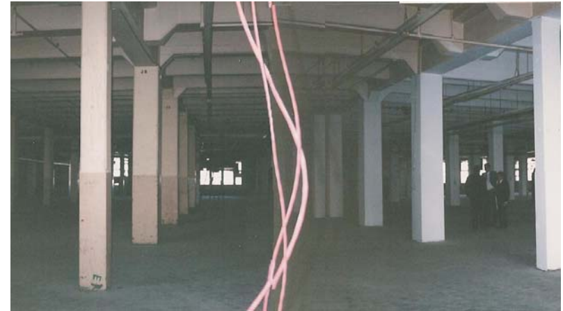
View of an un-renovated floor of the Center 3 Building
