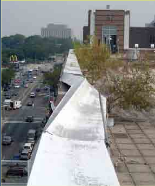
Hostos CC: roof parapet of 450 Grand Concourse bldg
