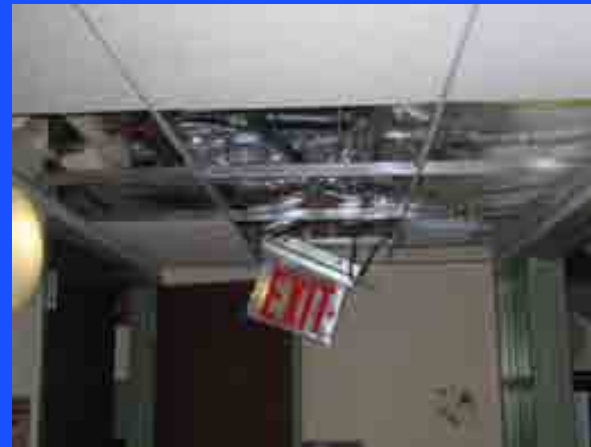
Queens College: stairway exit
