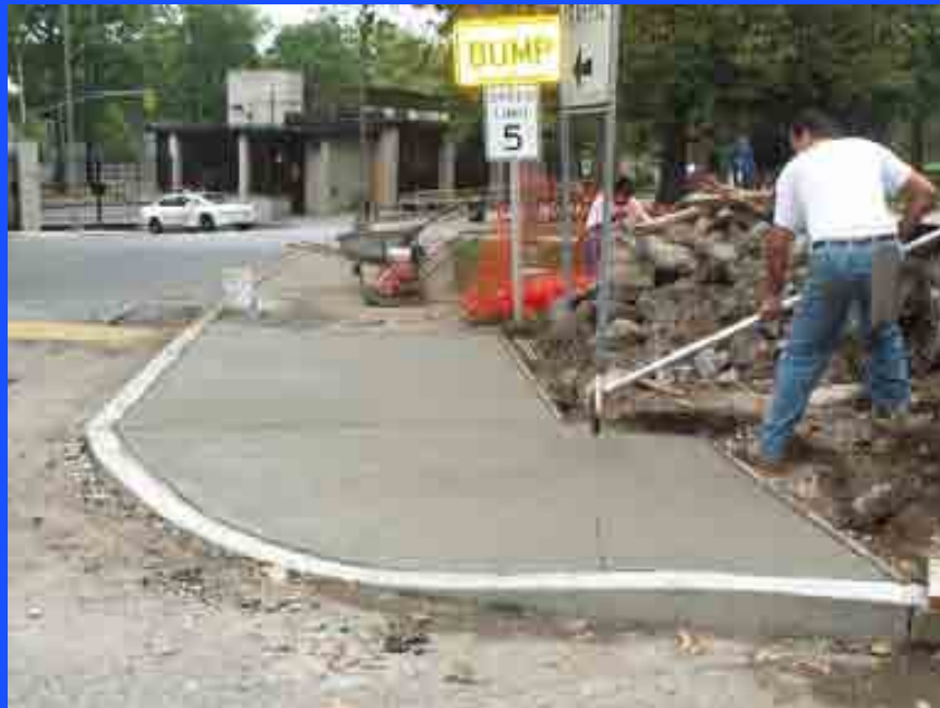
construction of ADA curb cuts
