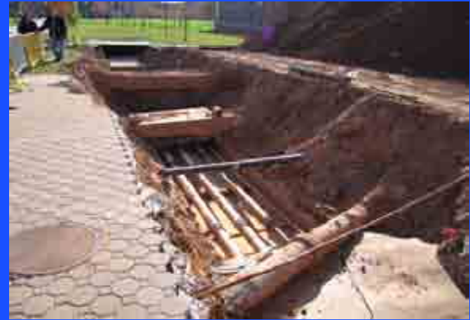
CSI: repair of heating / hot water pipes
