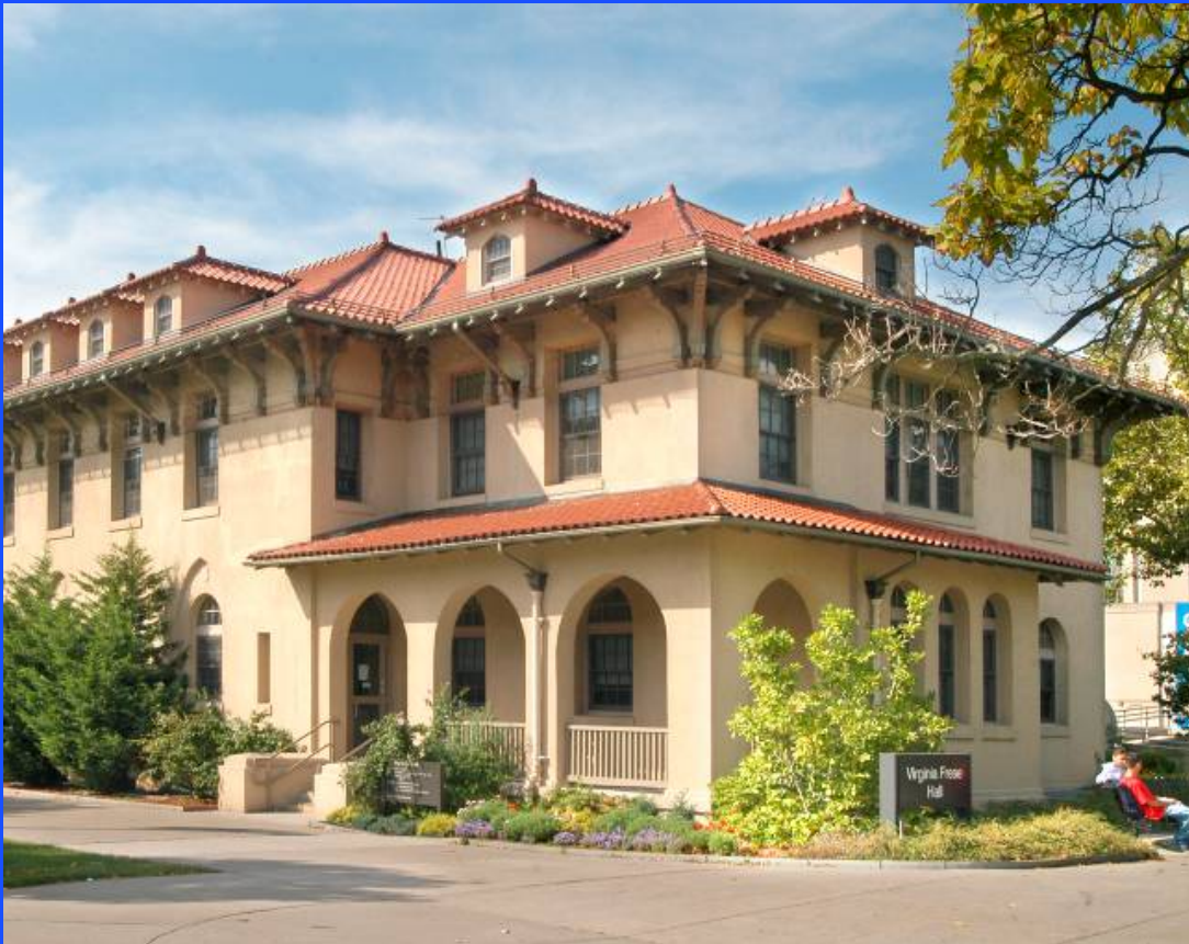
Queens College: Frese Hall Renovation
