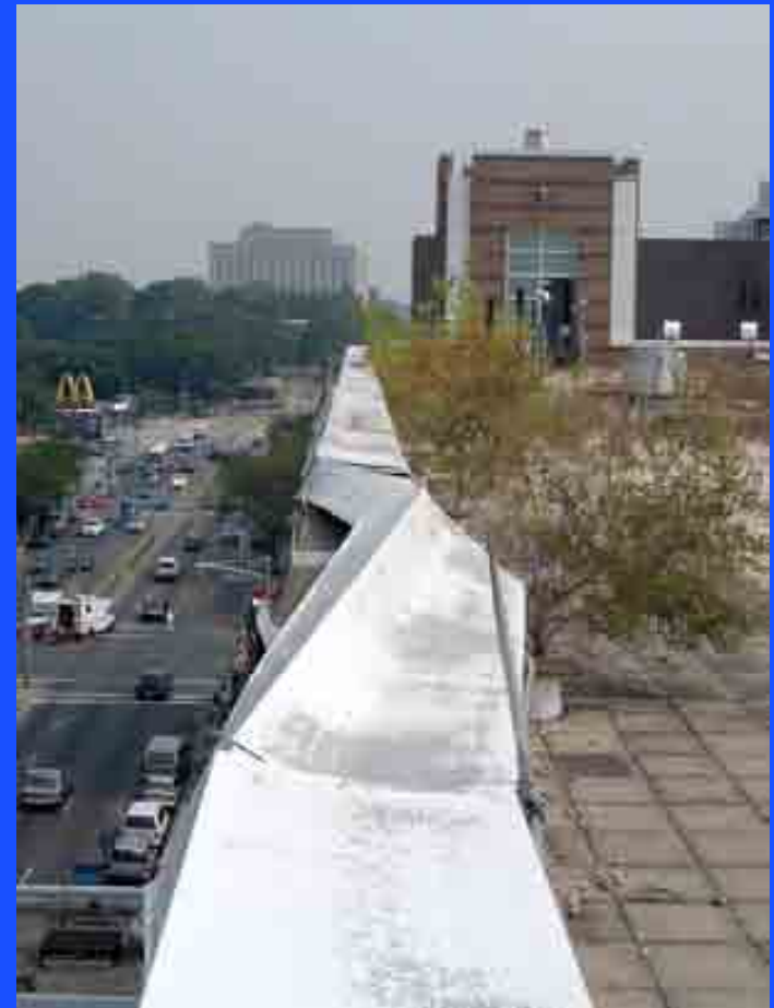
Hostos CC: building parapet
